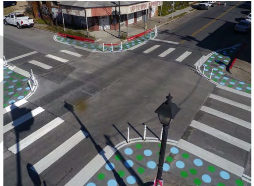
Figure 90. Testing intersection bump outs in community streetscapes can be done with paint (Austin example from bloomberg.com)
