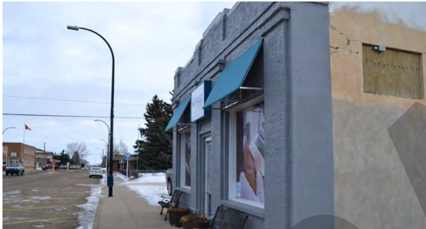
Figure 42. The lights on Main Street are not designed to create a comfortable environment for pedestrians
