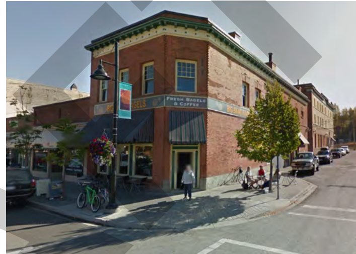
Figure 72. Intersection with gathering areas in bump outs in Fernie BC (image from Google Maps)
