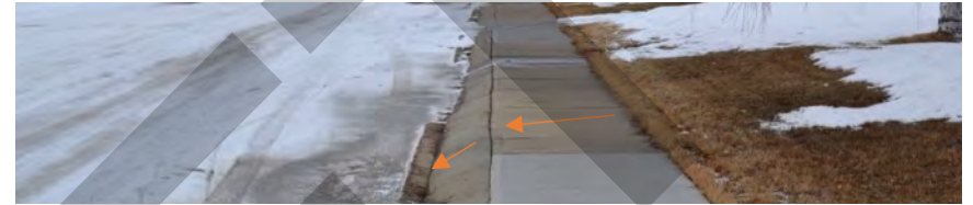
Figure 30. Sloped curbs can direct wheeled mobility devices into the street if the sidewalk is also sloped
