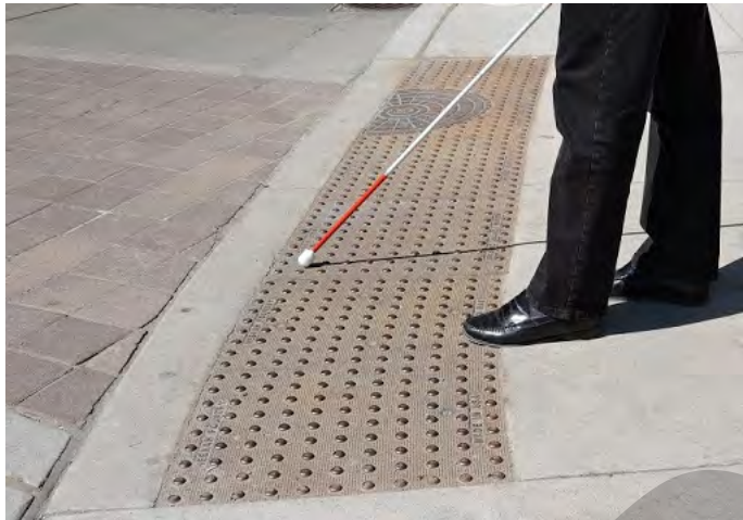
Figure 84. Tactile indicator mat provides warning of imminent intersection crossing.
