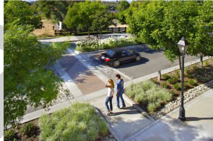
Figure 82. Raised crosswalk; this image shows different paving materials to emphasize the pedestrian zone. Painted pavement can achieve a similar visual effect.
