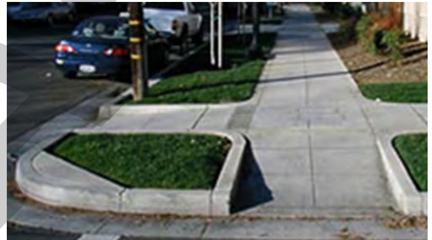
Figure 88. Curb cuts should be in line with the path of travel, one for each sidewalk.
