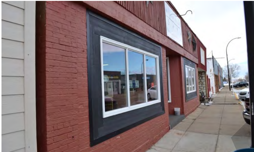
Figure 35. Building frontages directly adjacent to the sidewalk create an appealing pedestrian experience
