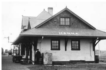
Hanna's Train Station in 1913. It has since been renovated and serves as the community Visitor Information Centre
